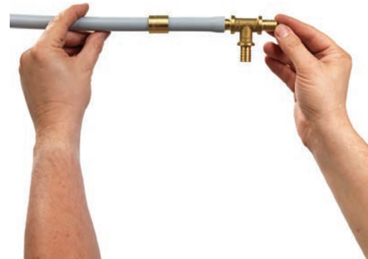
▲ Fig. 23: Push the fitting into the pipe. After a short period of time, the fitting has a tight fit in the pipe.
